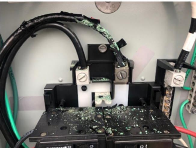
Photo 14: Failure to torque the lugs to the manufacturers specification: NEC 110.14(D)
